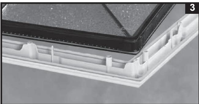
Position the frame square within the aperture, then place the glass gently on to the outer cassette (Glass units must be 1" thick or 26mm). Ensure the seal is secure to the glass.
